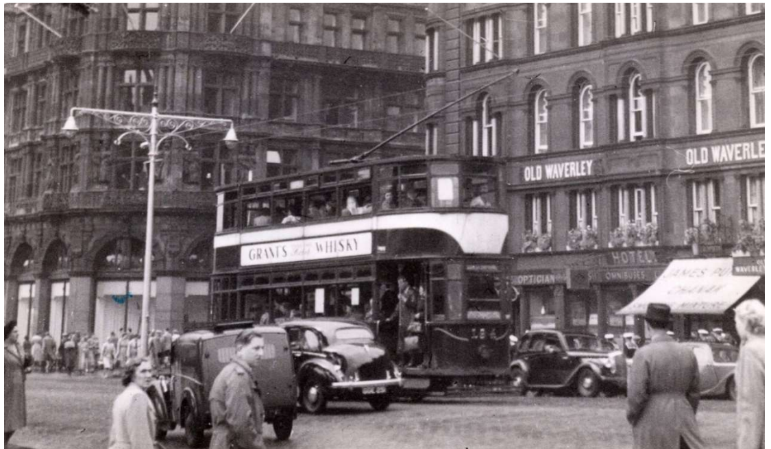
Tram at the east end of Princes Street, 1956.
