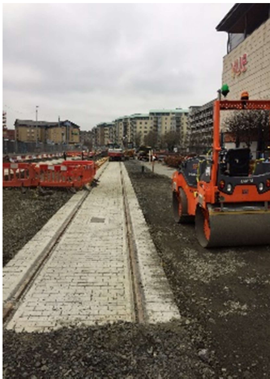
Tramworks at Ocean Terminal.
